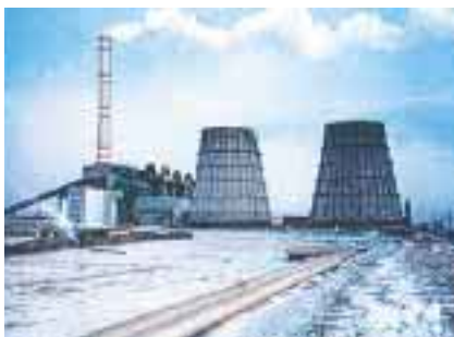
Rehabilitation Project of the 4th Thermal Power Plant in Ulaanbaatar
