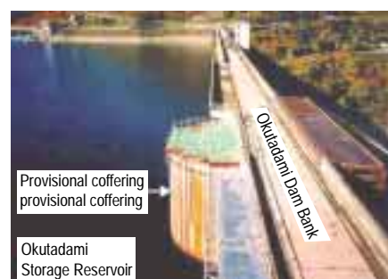
Provisional coffering, Okutadami Dam
