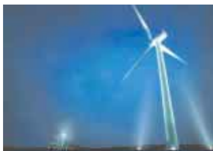
Tokyo Bayside Wind Power Plant (Tokyo)
