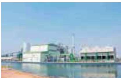
Roi-Et Hull-fired Thermal Power Station
