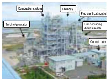
Full view of test unit for power generation technology using RDF
