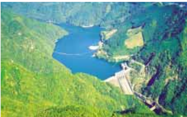
Sakuma Power Station (Shizuoka Prefecture)
