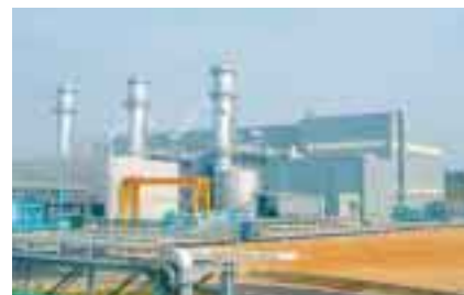
Chiahui Gas-Fired Power Station
