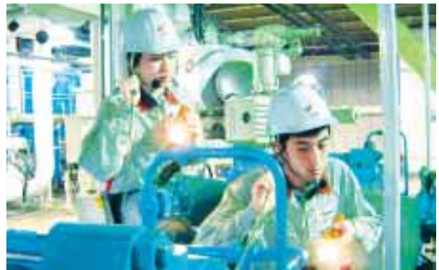
Audible inspection of pumps (Isogo Thermal Power Station)
