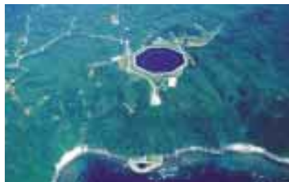
Demonstration test on sea water pumped storage power generation
