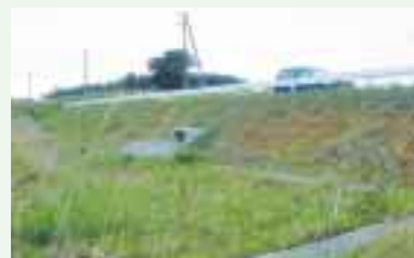
Covered crossing conduits below the road (for small animals to move)
