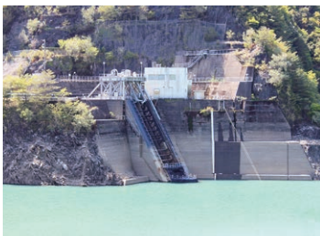
Surface water intake equipment (Yanase Dam, Kochi Prefecture)
