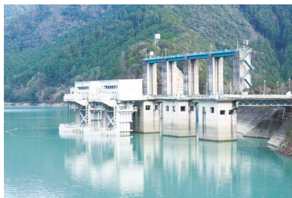
Surface-water intake equipment (Ikehara Dam, Nara Prefecture)
