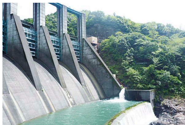
River maintenance discharge (Nanairo Dam, Mie and Wakayama Prefectures)
