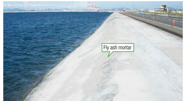
Surface lining of industrial waste landfill site using fly ash mortar *2 (J-POWER Hibikinada Waste Disposal Site No. 3, Kita-Kyushu)
