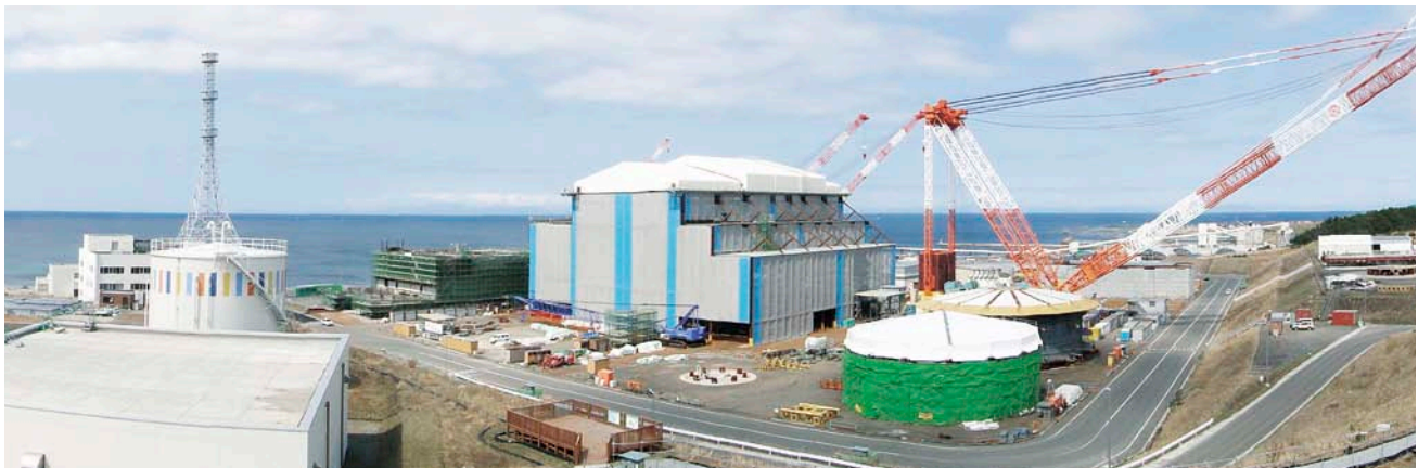
Status of construction of Ohma Nuclear Power Station (Spring 2012)
