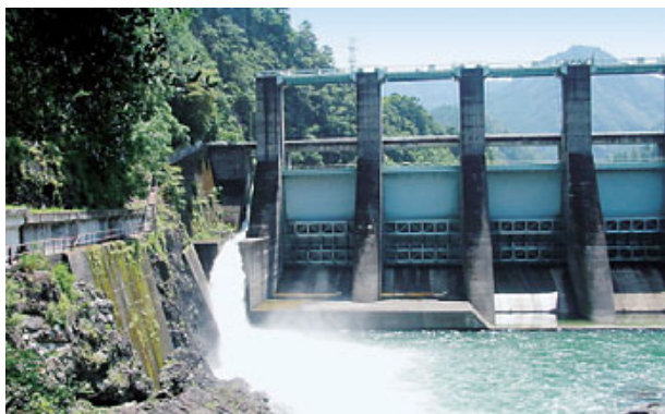
River maintenance discharge (Komori Dam, Mie Prefecture)
