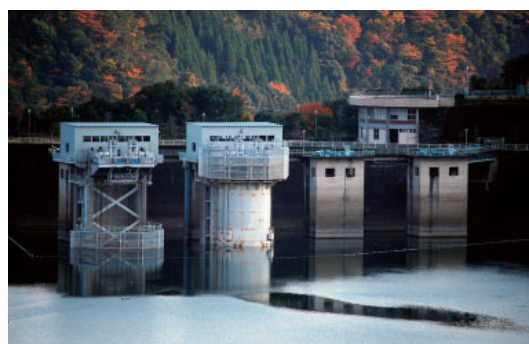
Surface-water intake equipment (Ikehara Dam, Nara Prefecture)
