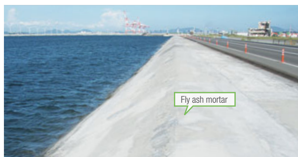
Surface lining of industrial waste landfill site using fly ash mortar (J-POWER Hibikinada Waste Disposal Site No. 3, Kita-Kyushu)
