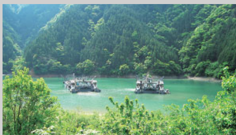
Dredger (Sakuma Dam Shizuoka and Nagano Prefectures)
