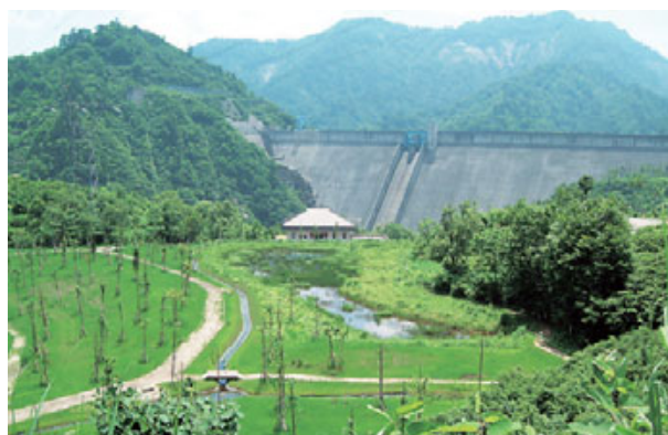
Restored wetlands, Okutadami Power Station
