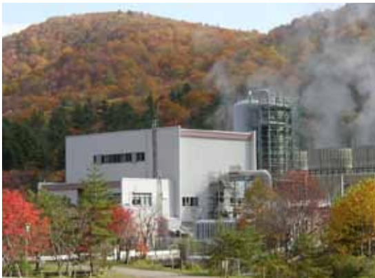
Onikobe Geothermal Power Station (Miyagi Prefecture)
