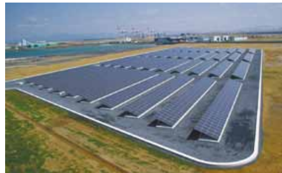
Hibikinada Solar Power Station (Kitakyushu)
