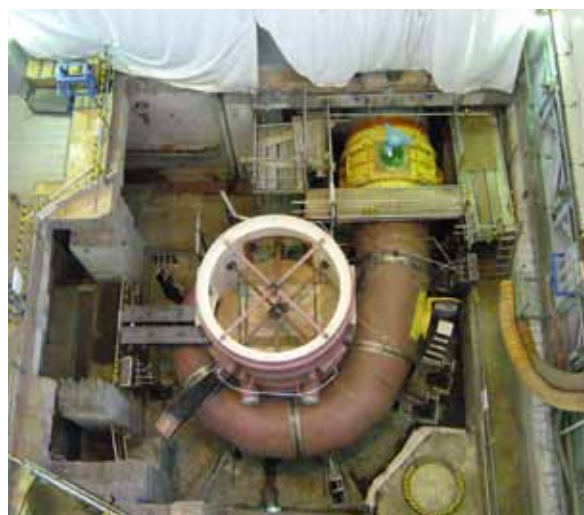
Replacement of key system components at Nukabira Power Station (Hokkaido)
