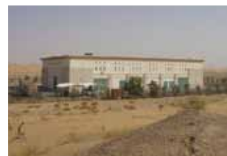
District cooling project, United Arab Emirates
