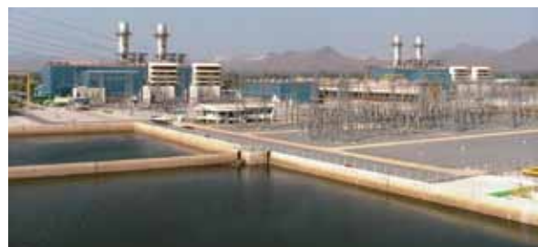
Kaeng Khoi 2 Gas-Fired Thermal Power Station (Thailand)
