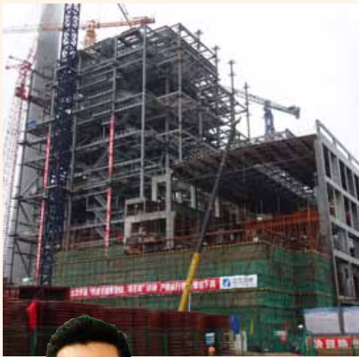
Xinchang Coal-Fired Thermal Power Station under construction (China)
