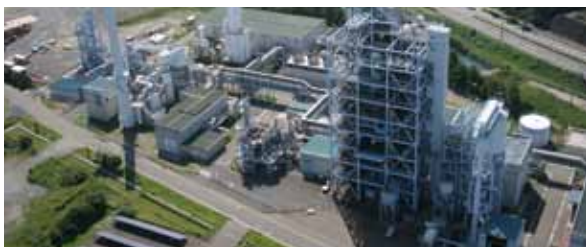
EAGLE pilot plant (Kitakyushu)
