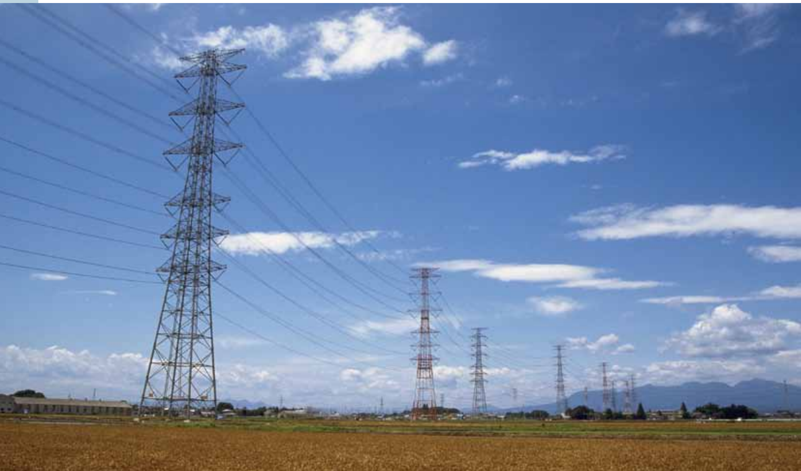
Tadami Main Transmission Line (Gunma Prefecture)
