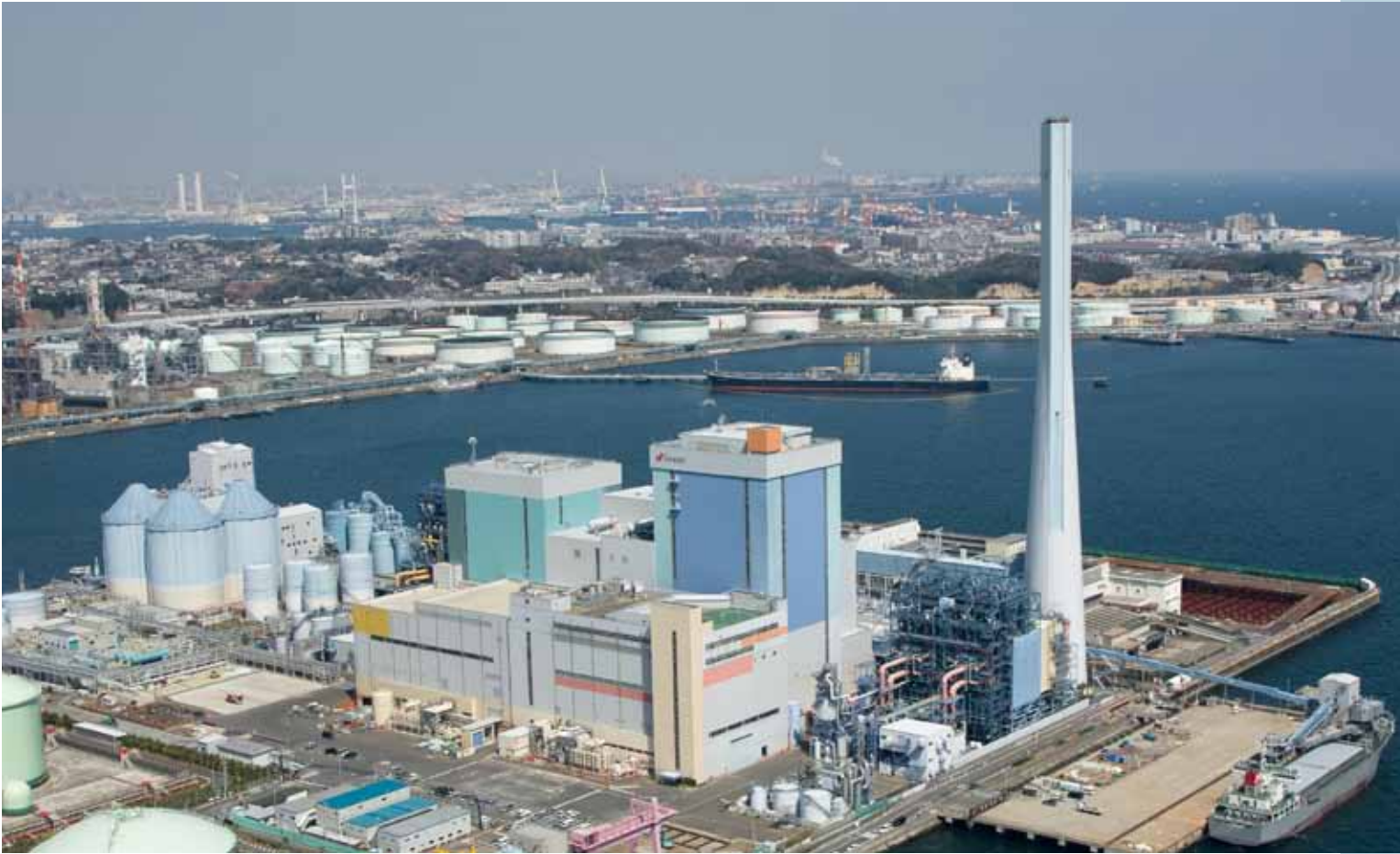
Isogo Thermal Power Station (Yokohama)
