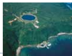
Okinawa Yanbaru Seawater Pumped Storage Power Station
