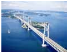
Honshi Interconnecting Line
