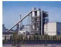
Itoigawa Power Station (IPP)
