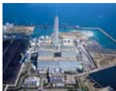
Matsuura Thermal Power Station
