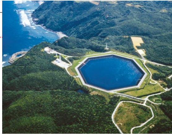
Okinawa Yanbaru Seawater Pumped Storage Power Station
