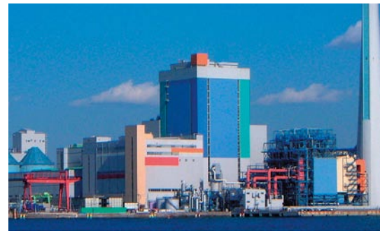
Isogo Thermal Power Station
