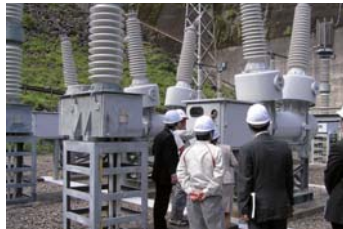
Kouchi Power Administration Office (Kochi Prefecture)
