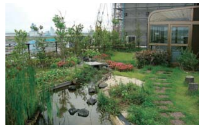
Rooftop garden at the J-POWER Wakamatsu Research Institute
