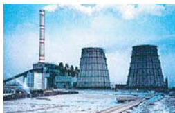
Rehabilitation Project for the Fourth Thermal Power Plant in Ulaanbaatar (Mongolia)
