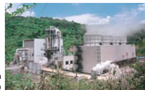
Onikobe Geothermal Power Station (Miyagi Prefecture)
