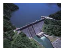
Tagokura Dam and Tagokura Power Station (Fukushima Prefecture)
