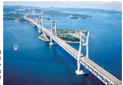
Power cables are laid across the Seto Ohashi Bridge, creating the Honshu Interconnecting Transmission Line linking Honshu and Shikoku.
