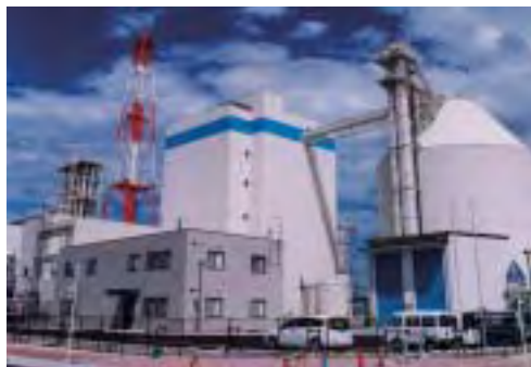
Omuta Recycle Power Station (unconsolidated affiliate) Omuta, Fukuoka Prefecture; startup December 2002 This RDF (refuse-derived fuel) power plant generates electricity efficiently using MSW ♻️ as fuel.
