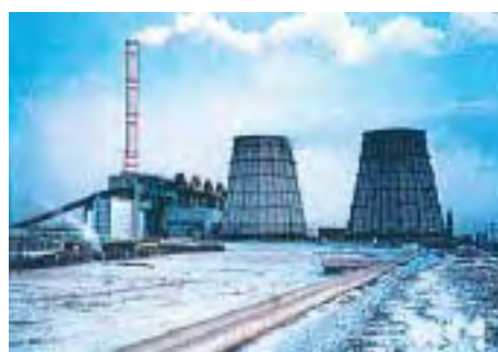
Ulaanbaatar Fourth Thermal Power Plant Rehabilitation Project (Mongolia)
