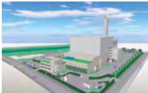
Narumi Waste Disposal Plant, Nagoya (unconsolidated affiliate) Nagoya, Aichi Prefecture; startup (planned) July 2009 This project for waste-power generation using a gasification and melting system will not only generate electricity from MSW (thermal recycling) but also recycle materials for reuse.
