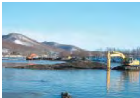
Sediment dredging at Senbiri Dam (Hokkaido Prefecture)
