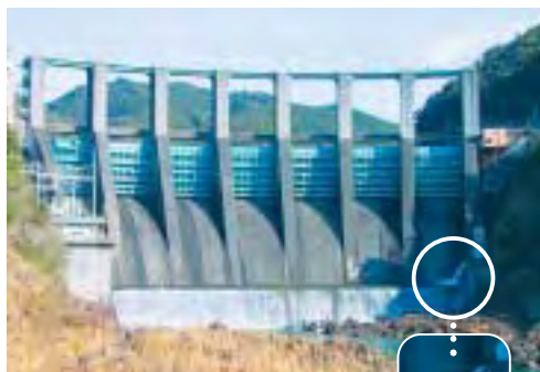
River maintenance discharge (circled area) at Nanairo Dam (Wakayama Prefecture/Mie Prefecture)
