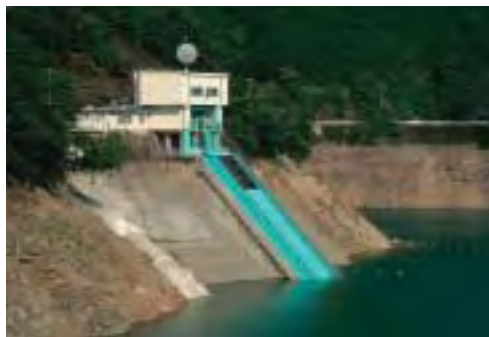
Sakamoto Dam surface-water intake system under construction (Nara Prefecture)
