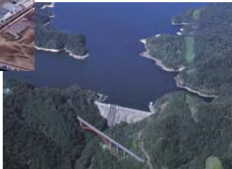
Nukabira Power Station (Hokkaido)
