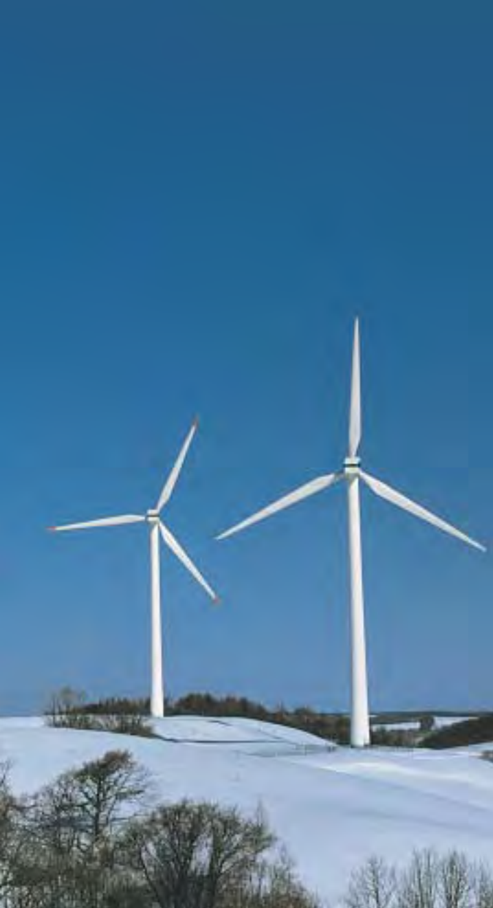
Tomamae Winvilla Power Plant (Hokkaido pref.)
