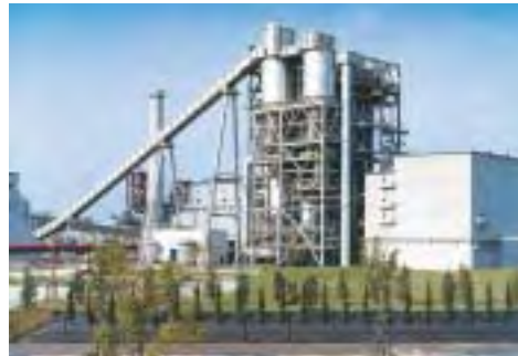
Itoigawa Power Station (Niigata Prefecture)
