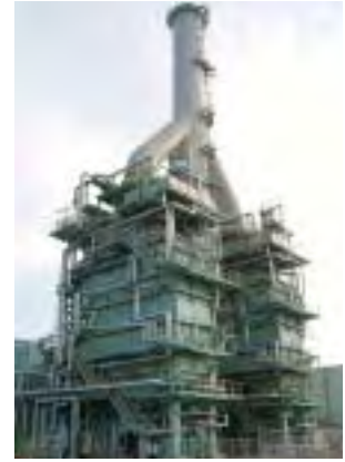
Ichihara Power's Ichihara Power Station (Chiba Prefecture)
