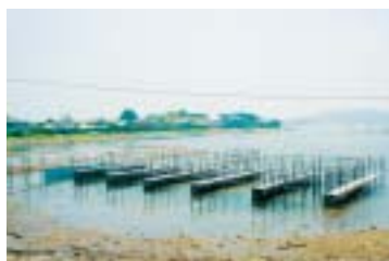
Demonstration test of technology to cleanse bottom mud.
