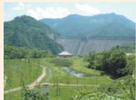
Site of wetland re-creation, Okutadami-Otori Hydro Project
