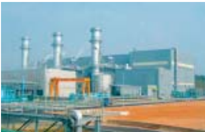
Chia-Hui Gas Combined-Cycle Power Generation Plant (Taiwan)
