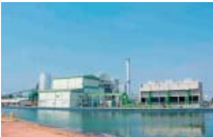
Roi-Et Rice-chaff-fired Thermal Power Generation Plant (Thailand)
