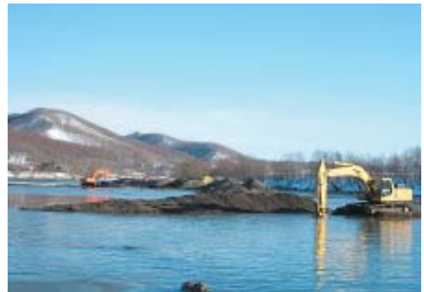
Sediment dredging at Senbiri Dam (Hokkaido Prefecture)
