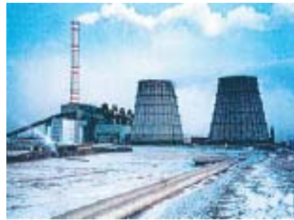
Rehabilitation project, 4th Thermal Power Plant, Ulaanbaatar (Mongolia)
