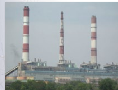
Bakreswar Thermal Power Station (India)
