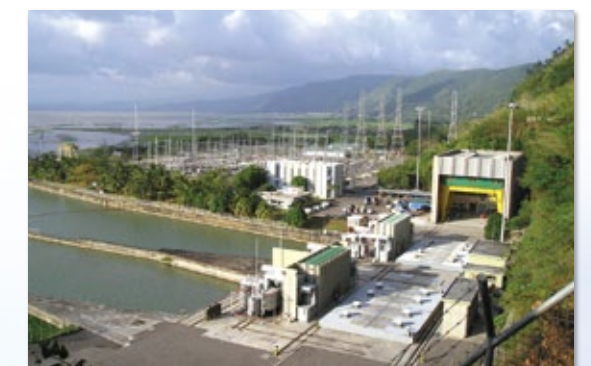
CBK (Kalayaan) Pumped Storage Power Station (The Philippines)
