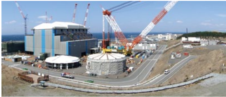
Ohma Nuclear Power Station under construction
