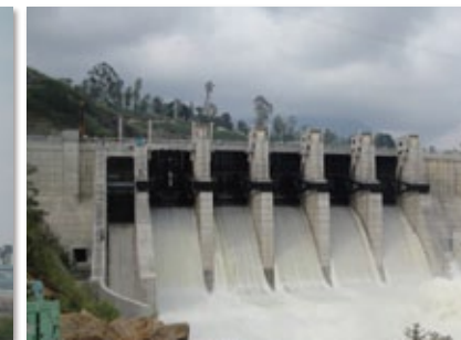
Upper Kotmale Hydroelectric Power Station (Sri Lanka)
