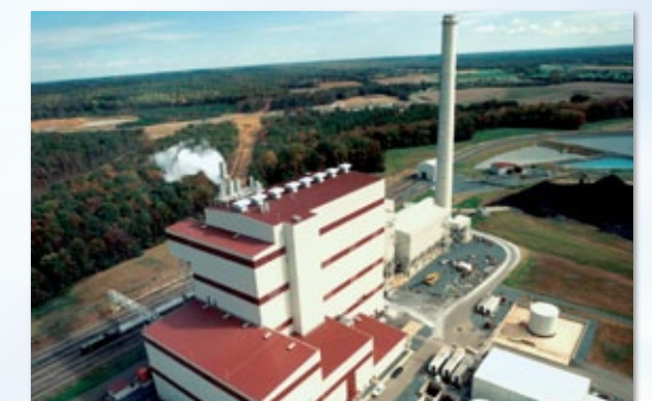
Birchwood Coal-fired Power Station (U.S.A.)
