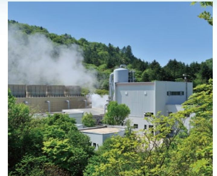
Onikobe Geothermal Power Station
