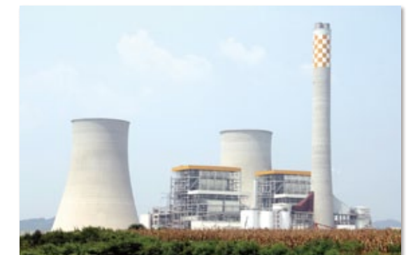
Hezhou Coal-fired Power Station (China)
