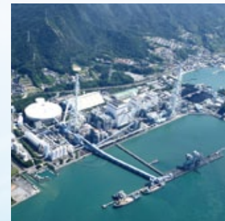
Takehara Thermal Power Station
