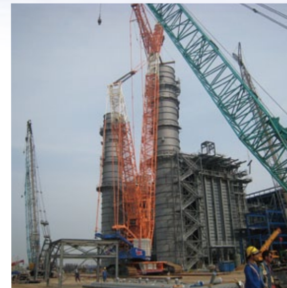
Utai Natural Gas-fired Combined Cycle Power Station (under construction in Thailand)
