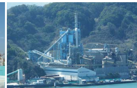
Tosa Power Plant
