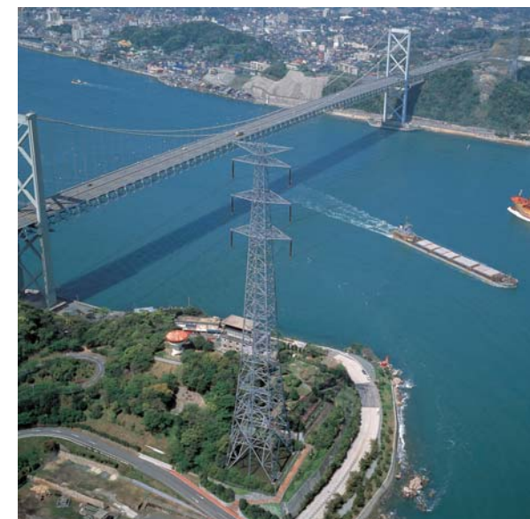
Kanmon Interconnecting Line
