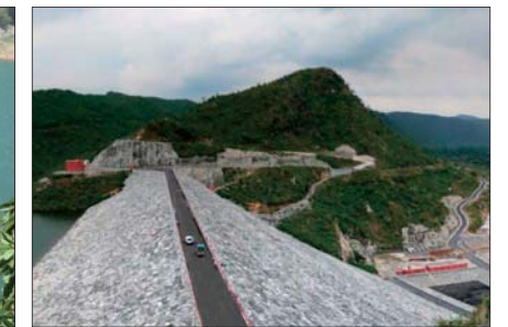
Purulia Pumped Storage Power Plant (India)
