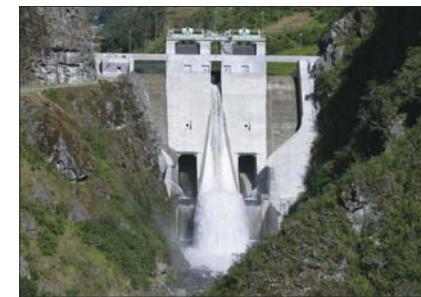
Yuncan Hydropower Plant (Peru)
