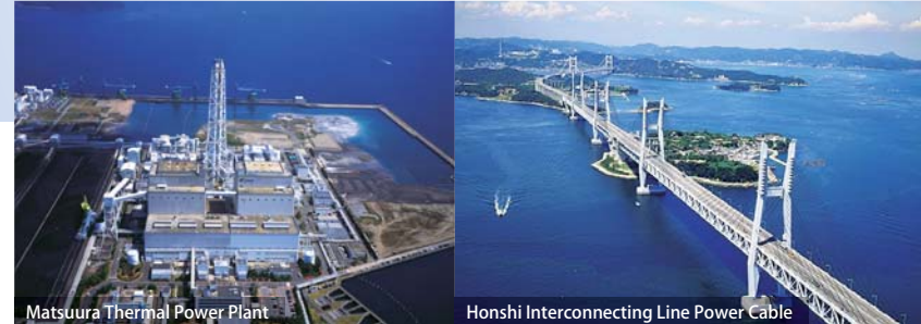
Matsuura Thermal Power Plant
