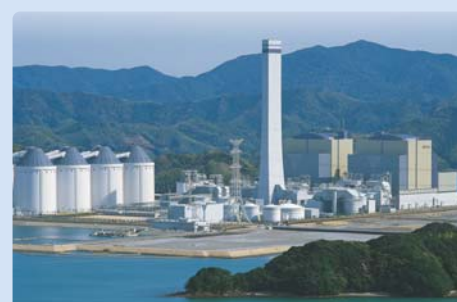
Tachibanawan Thermal Power Plant
