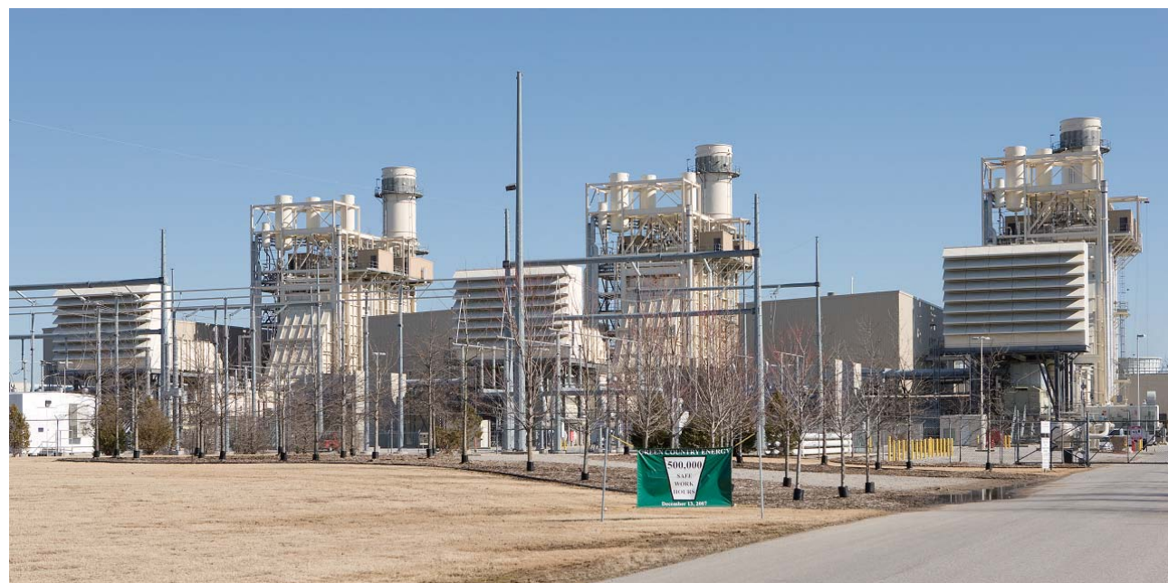
Green Country Thermal Power Plant (USA)
