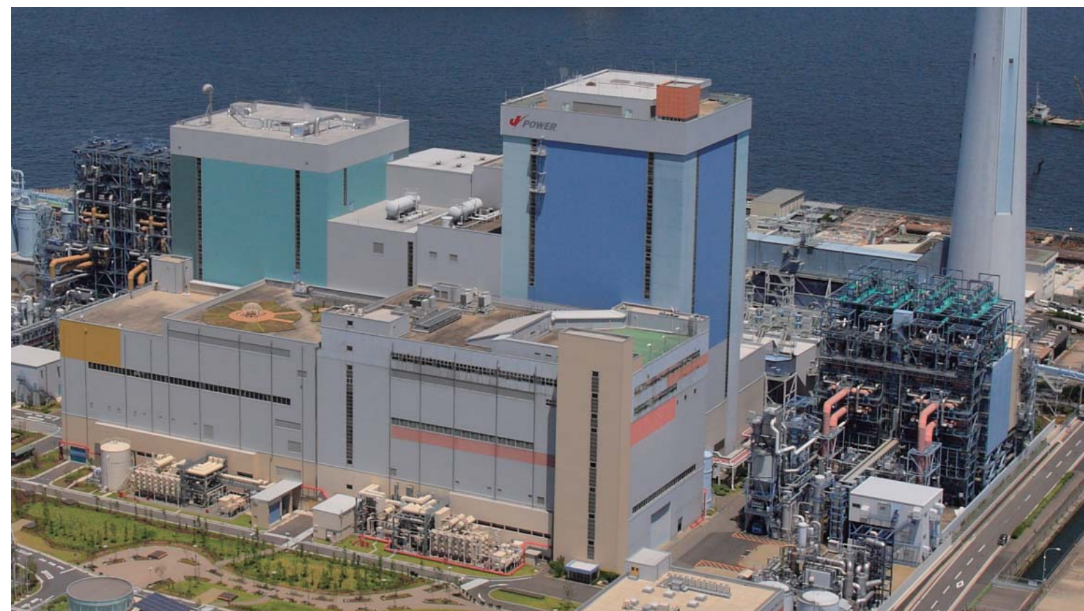
Isogo Thermal Power Plant
