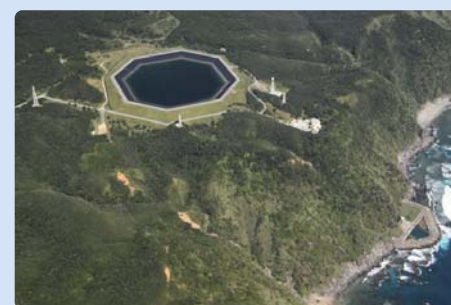
Okinawa Yanbaru Seawater Pumped Storage Power Plant
