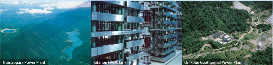
Numappara Power Plant
