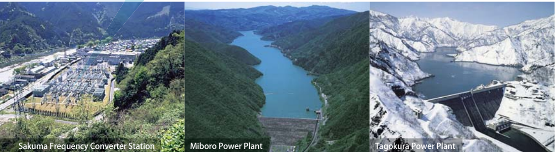
Sakuma Frequency Converter Station
