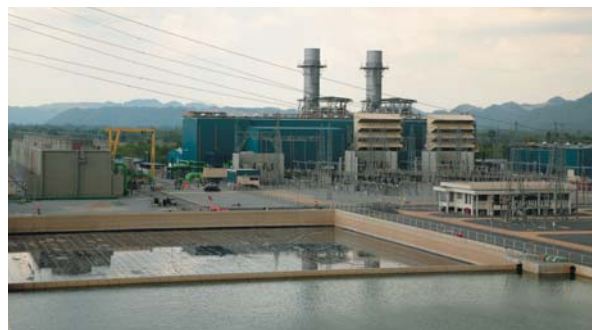
Kaeng Khoi No.2 Gas-Fired Thermal Power Plant (Thailand)
