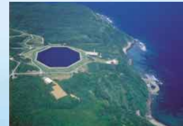
Okinawa Yanbaru Seawater Pumped Storage Power Plant
