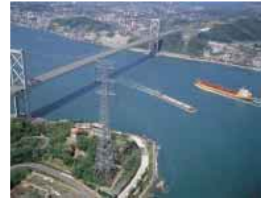
Kanmon Interconnecting Line
