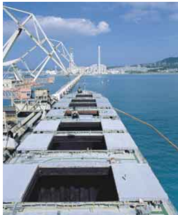
Coal Being Unloaded from a Collier Vessel at Ishikawa Coal Thermal Power Plant
