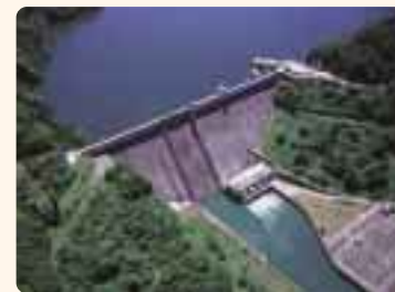
Concrete dam ( Tagokura Dam )
