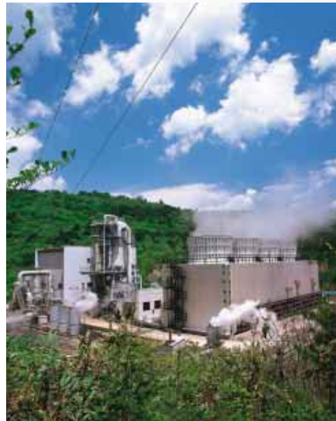
Onikobe Geothermal Power Plant
