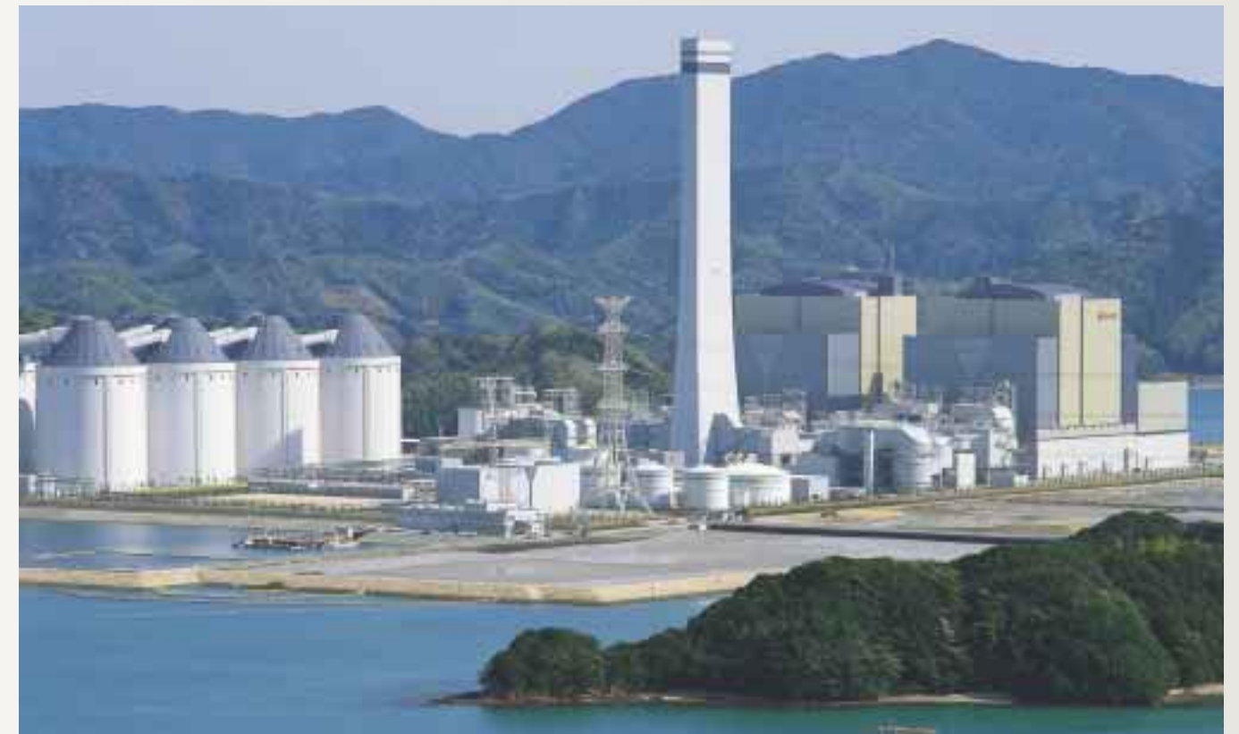
Tachibanawan Thermal Power Plant
