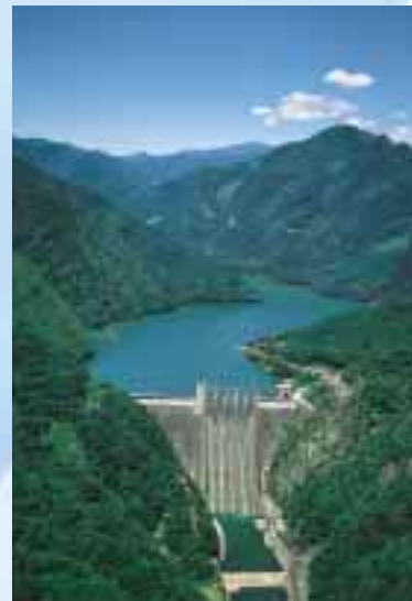
Sakuma Power Plant
