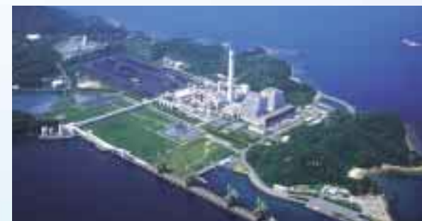
Matsushima Thermal Power Plant
