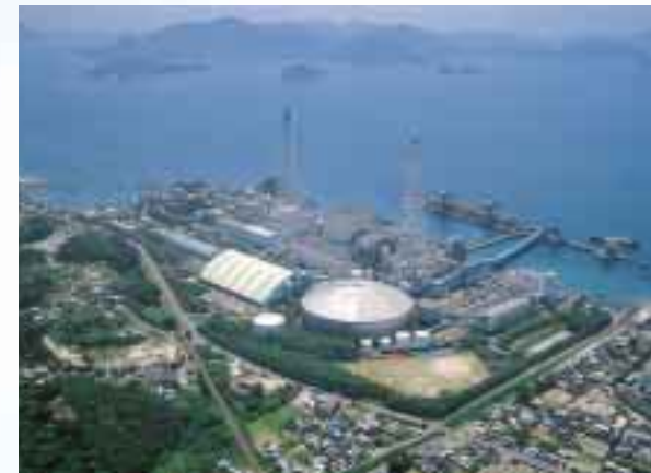
Takehara Thermal Power Plant
