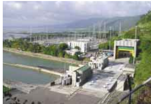
Kalayaan Pumped Storage Power Plant ( Philippines ) [ IPP ]
