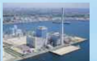
Isogo Thermal Power Plant
