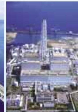
Matsuura Thermal Power Plant
