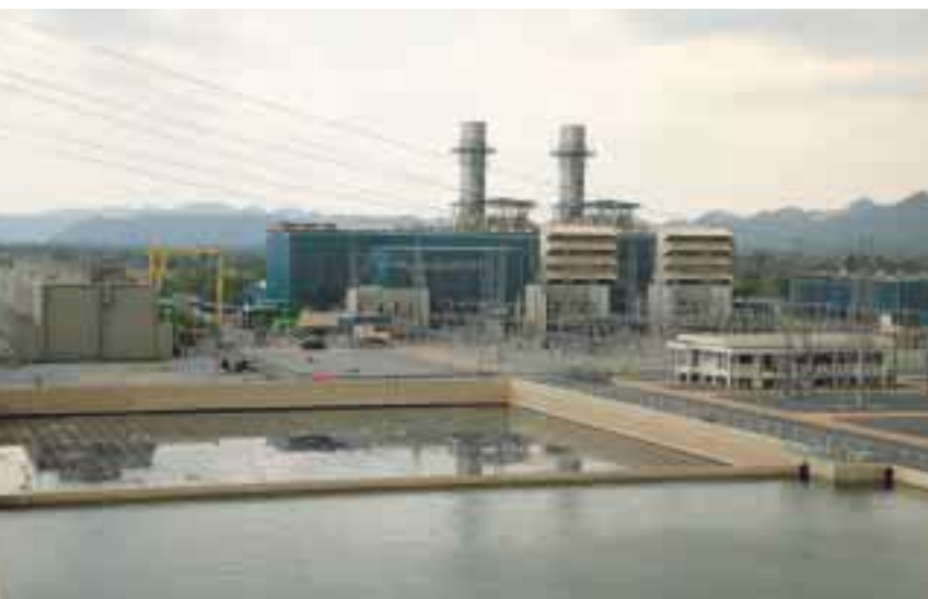
Kaeng Khoi No.2 Gas-Fired Combined Cycle Power Plant ( Thailand ) [ IPP ]
