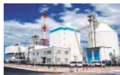
Omuta waste-fueled Power Plant
