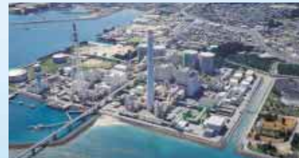
Ishikawa Coal Thermal Power Plant
