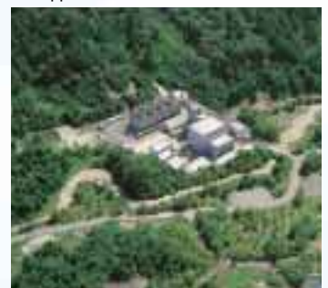
Onikobe Geothermal Power Plant
