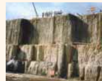
Earth retaining excavation work using ground improvement method employing coal ash
