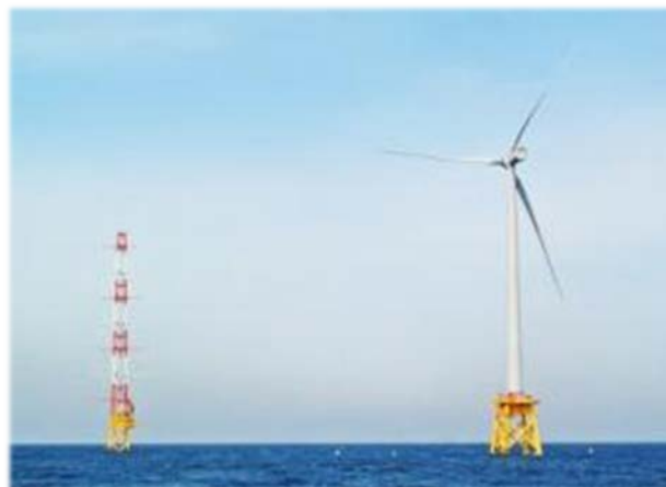
[洋上風力の取組み]
