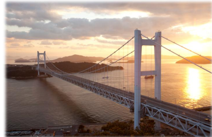
[Honshi Interconnecting Line]
