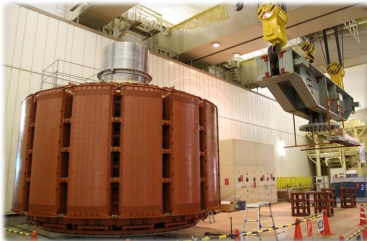
[Overhaul works at the Shimogou Power Plant]
