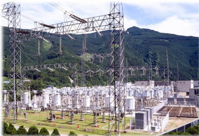
[Sakuma Frequency Converter Station]
