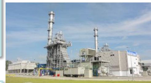
NK2 Cogeneration Power Plant in Saraburi, Thailand
