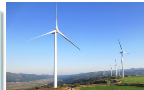
Kaminokuni Wind Farm
