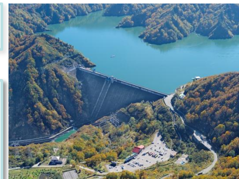
Okutadami Hydroelectric Power Plant
