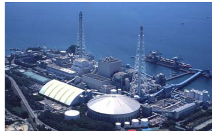
Takehara Thermal Power Plant
