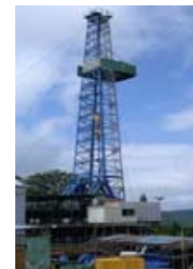
Exploratory Well Drilling
