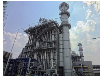
TLC (Mar. 2013, in operation)
