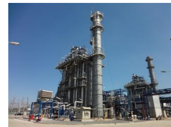
KP1 (Jan.2013, in operation)
