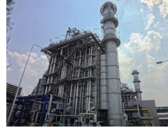
TLC (Mar. 2013, in operation)
