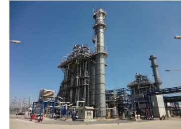
KP1 (Jan. 2013, in operation)
