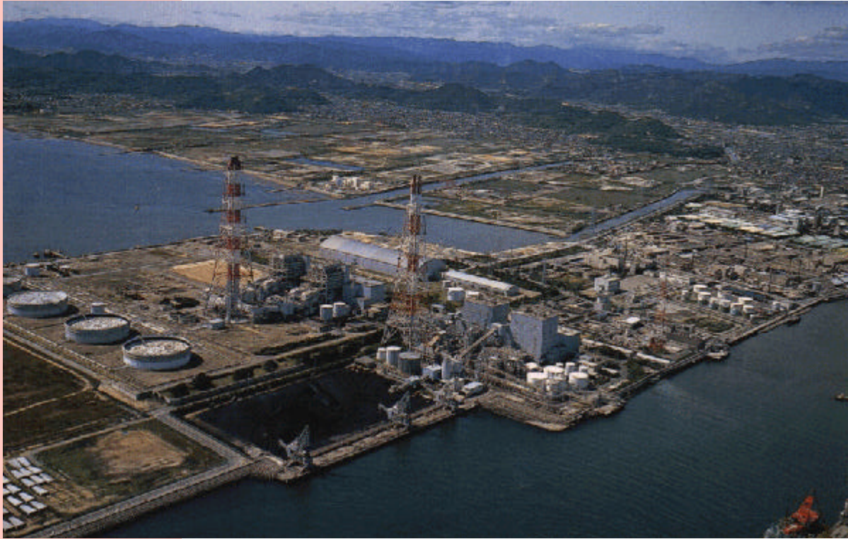
General View of the Project
