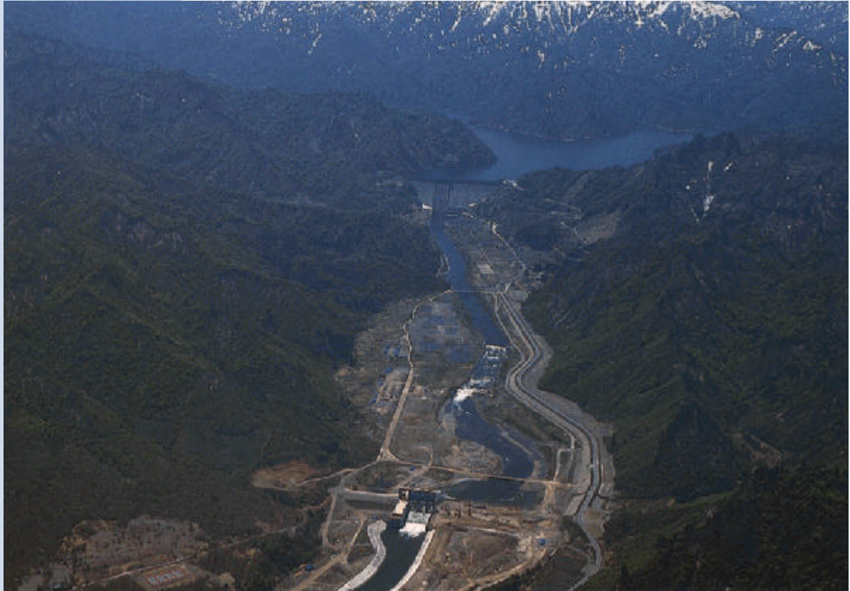
General View of the Project
