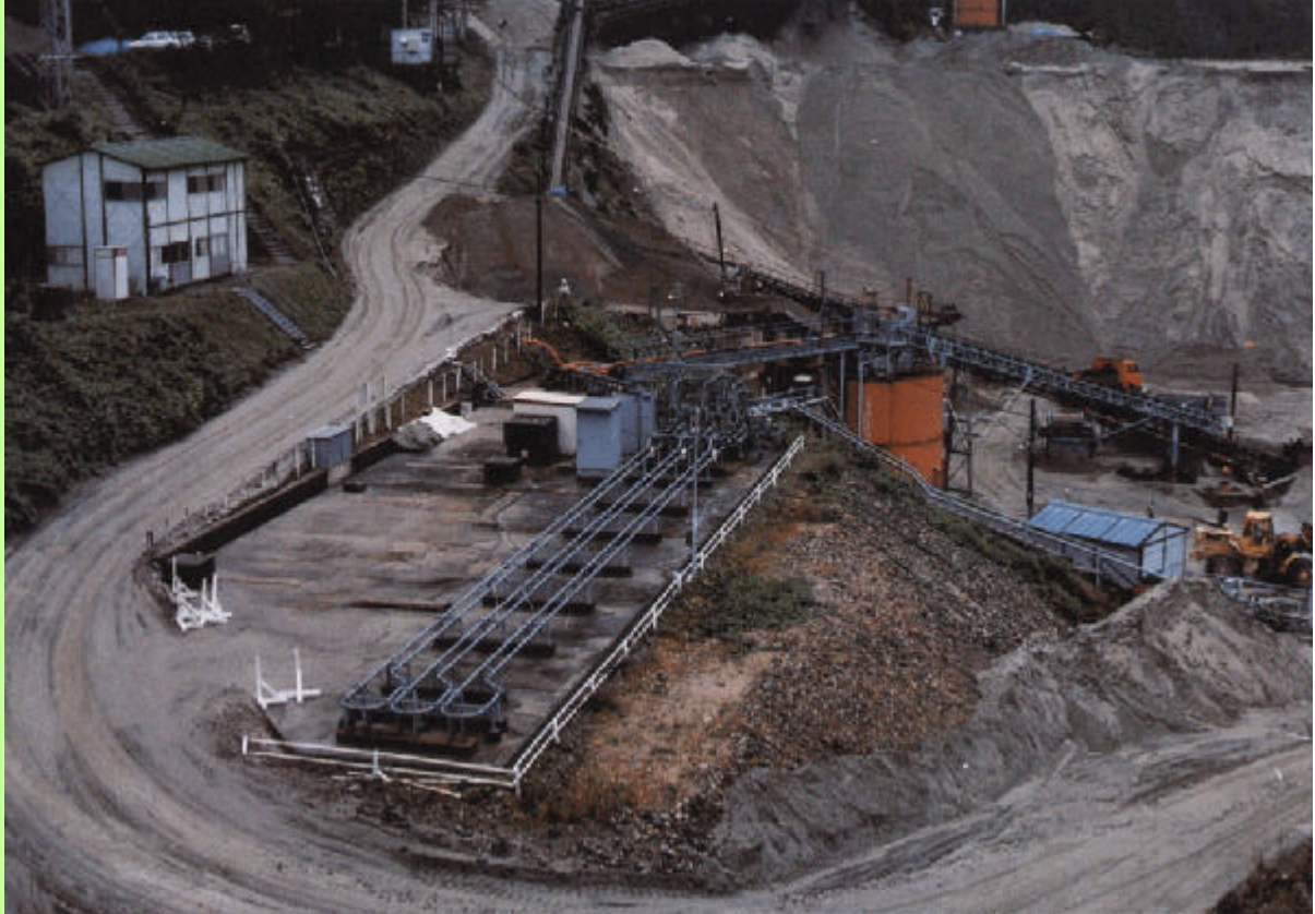
Sand Slurry Transported by Pipeline
