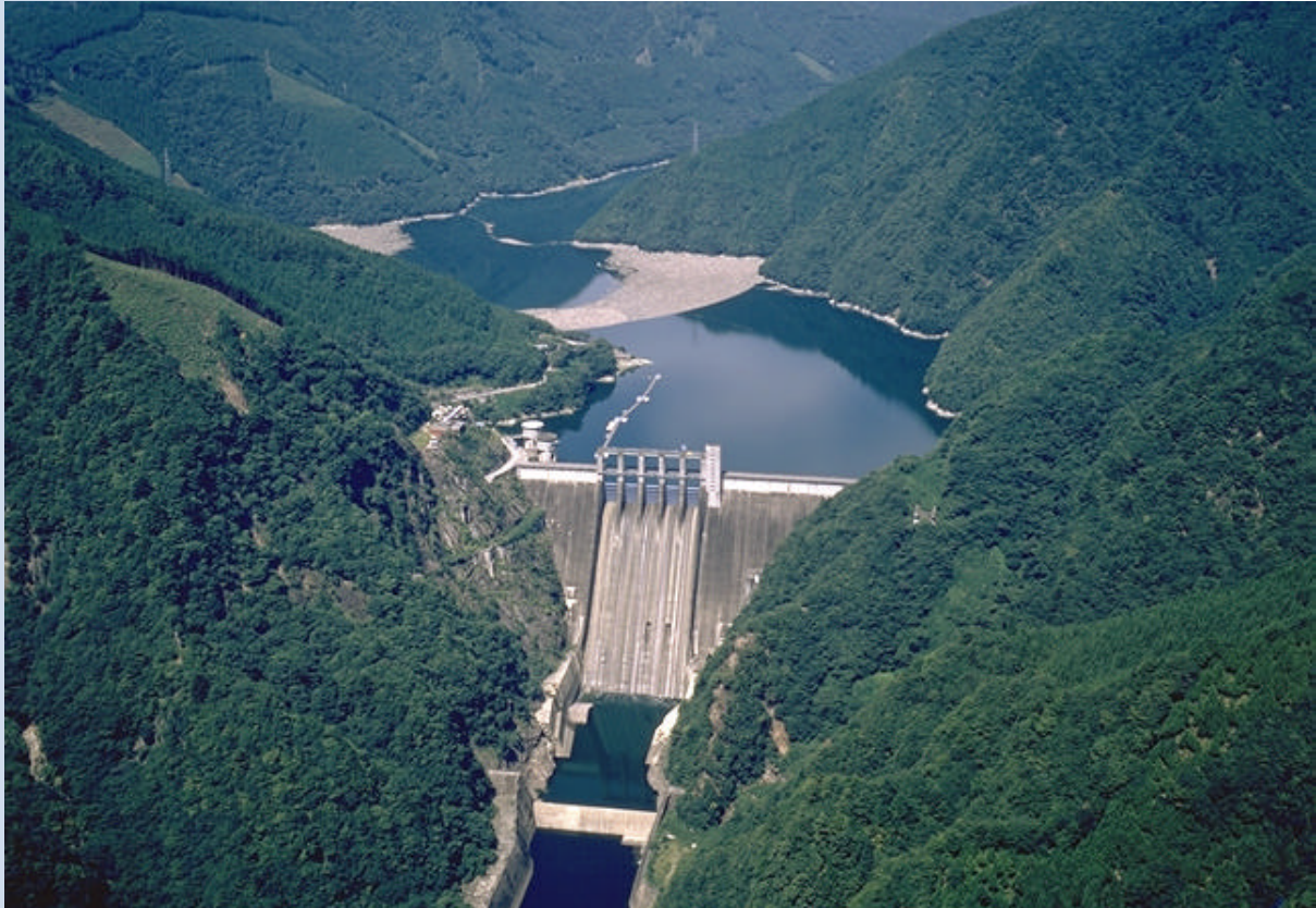
General View of Sakuma Dam
