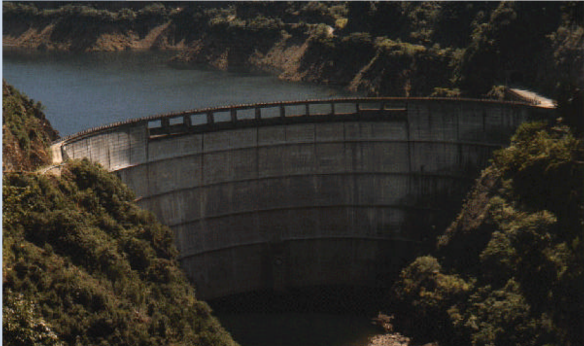
General View of the Project
