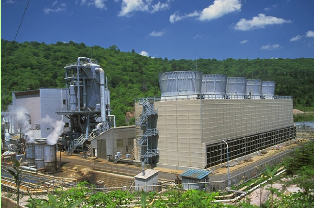
General View of Power Plant
