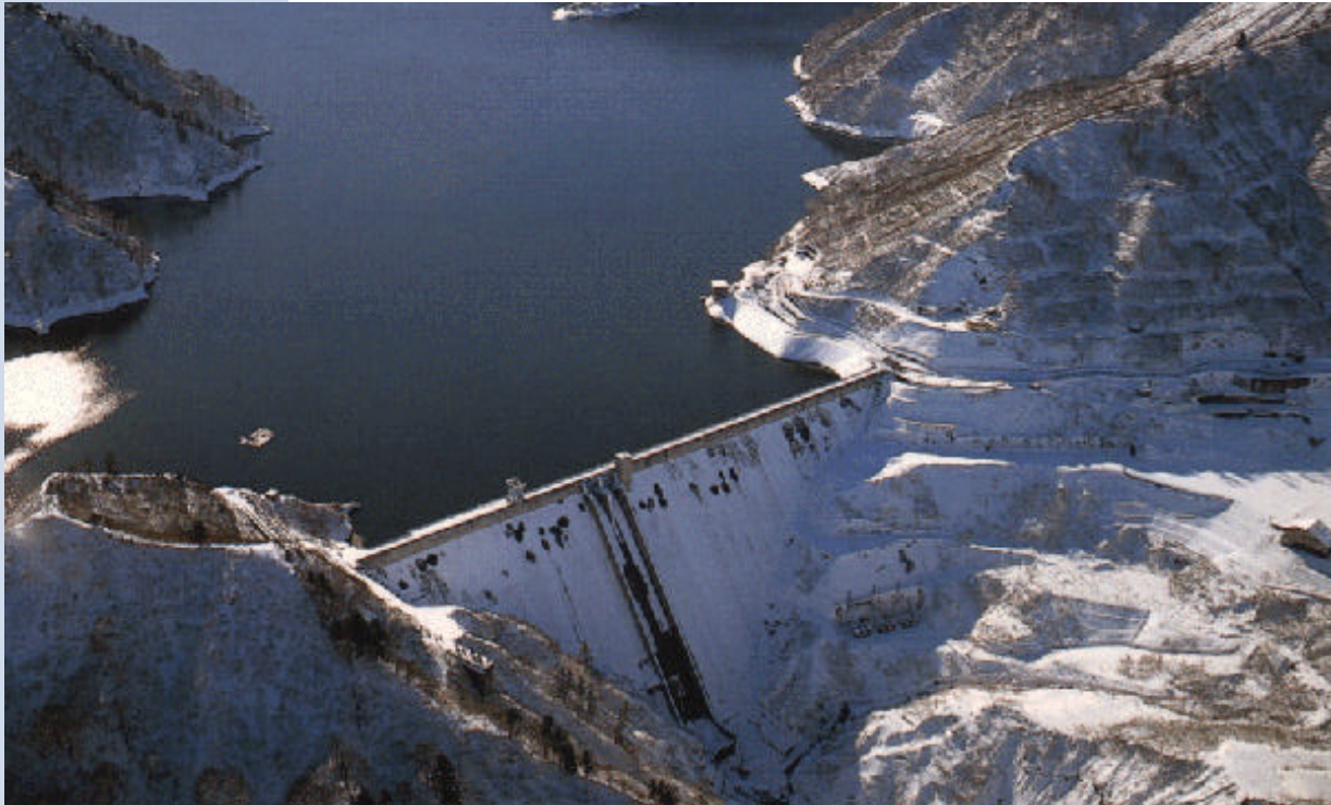
General View of the Project
