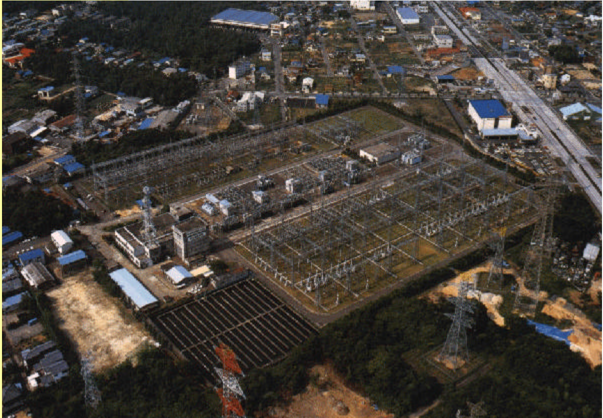
General View of Nagoya Substation
