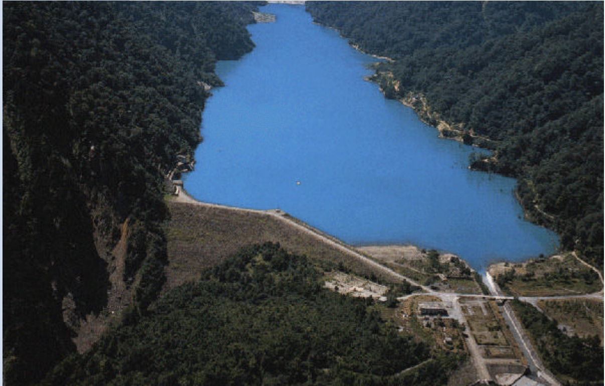
General View of the Project
