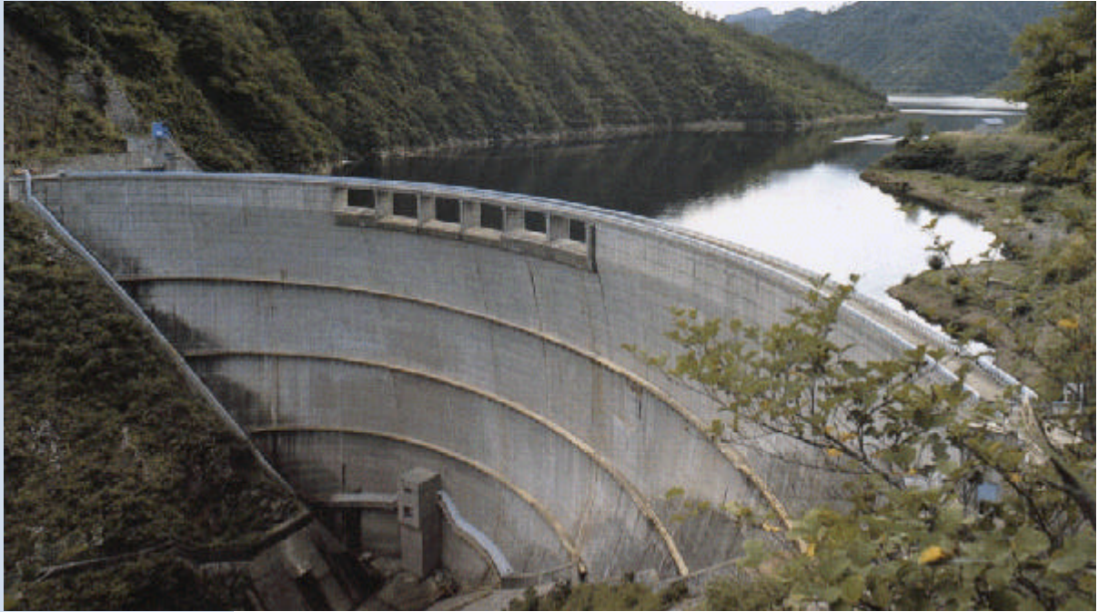
General View of the Project
