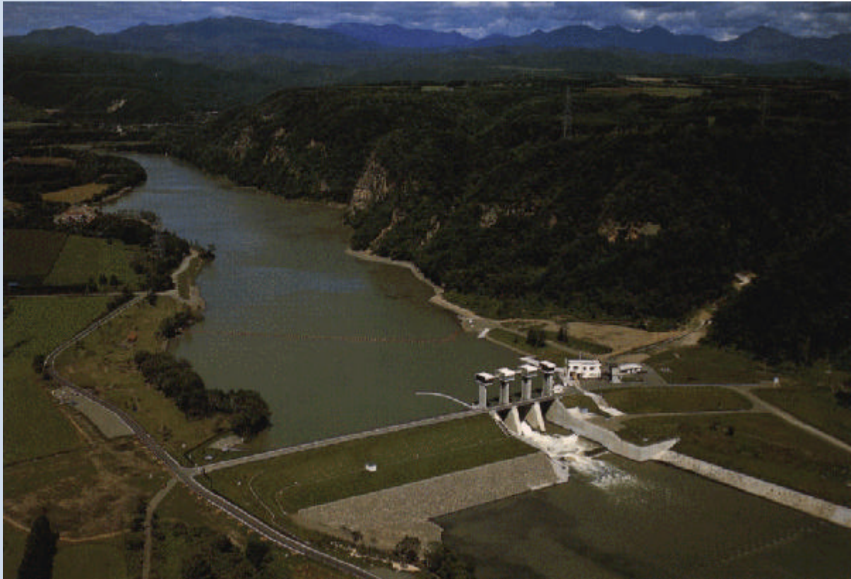
General View of Kuttari Dam
