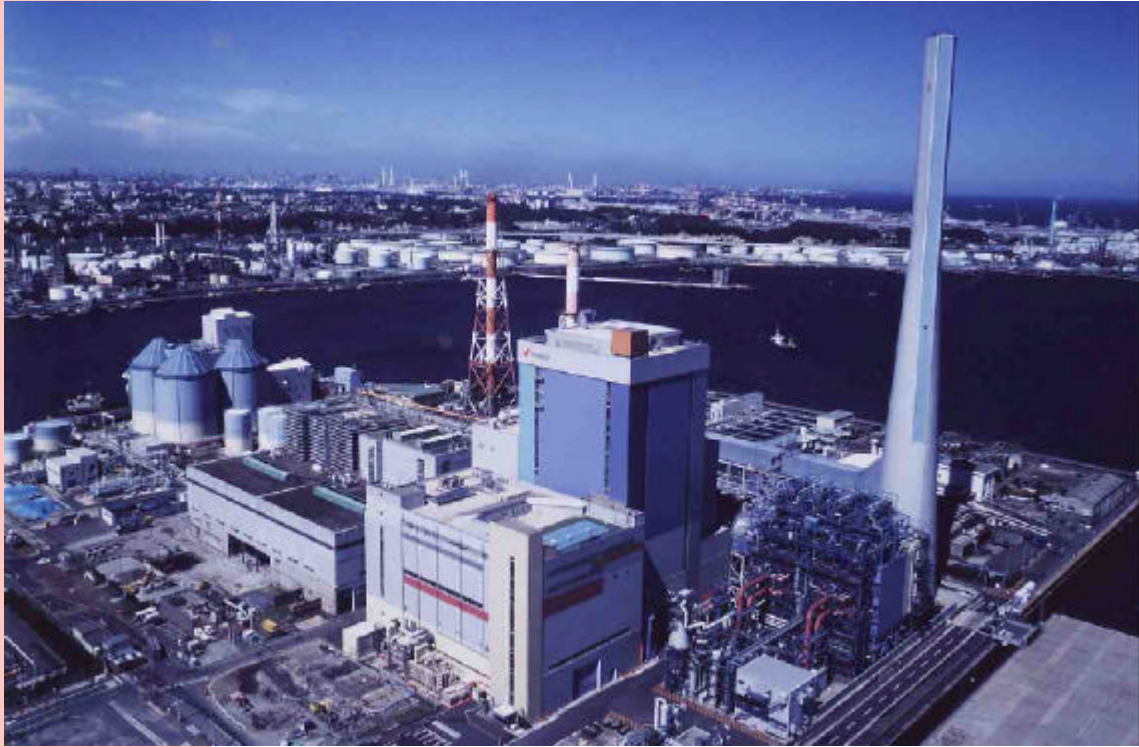
General View of the Project
