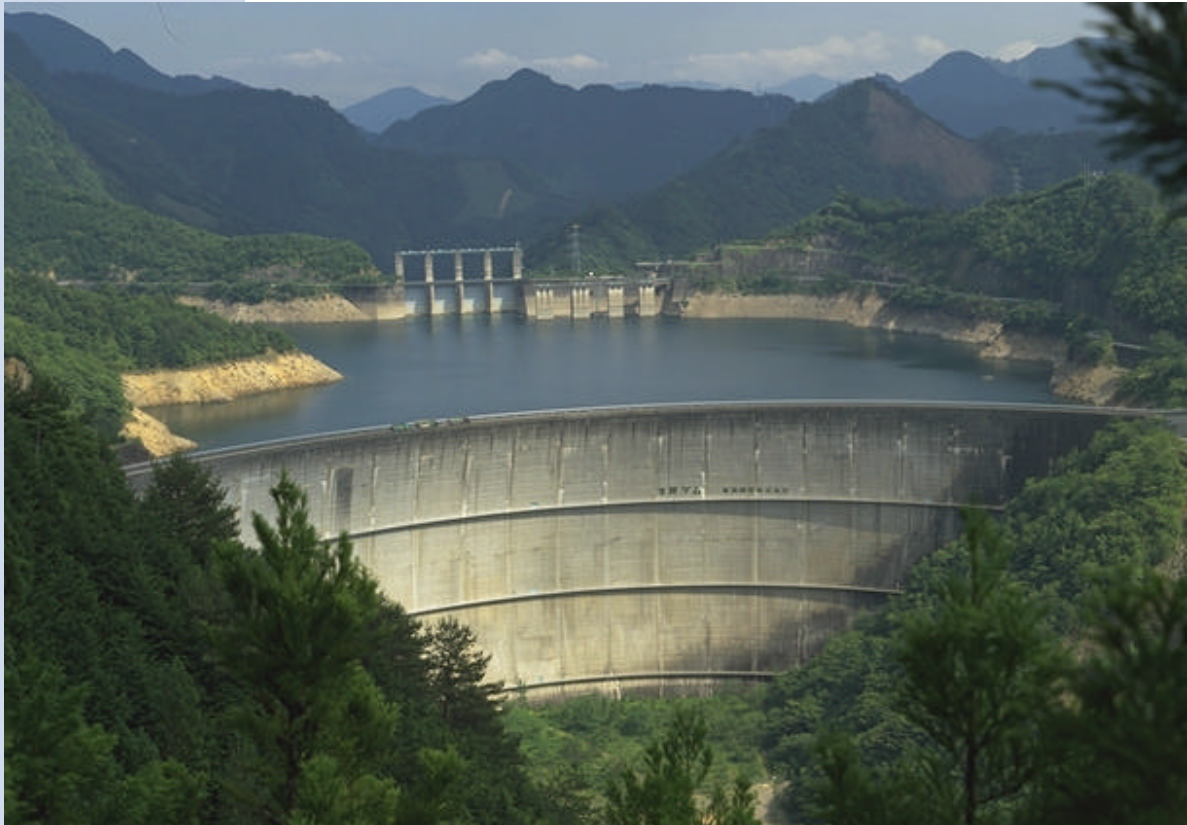
General View of Ikehara Dam
