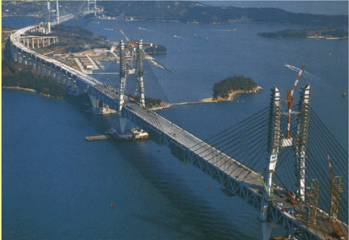
500kV OF Cables installed along with Seto-Ohashi Bridge.
