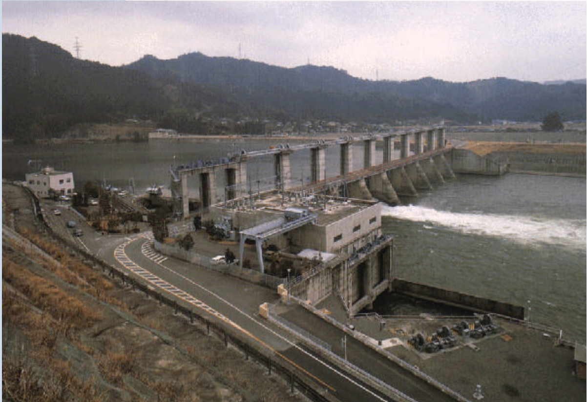
General View of the Project
