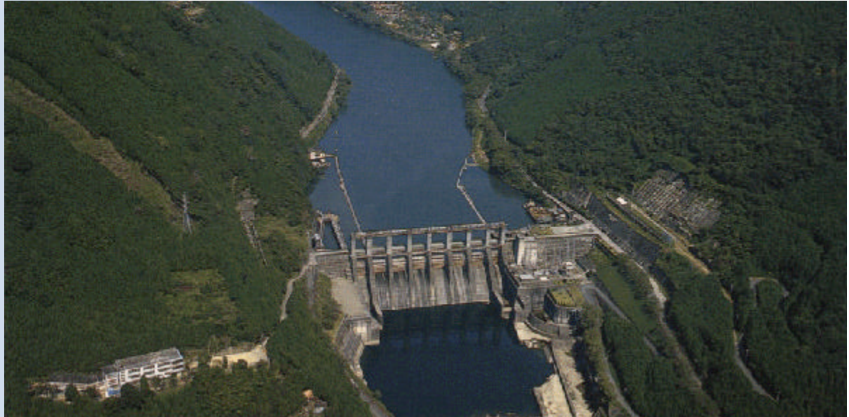
General View of Akiba Dam and Akiba No.2 Powerhouse
