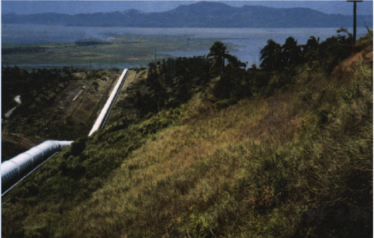
Project Site (Kalayaan Pumped Storage Power Station, 1st Stage)
