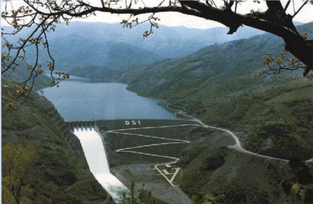
Operating Hasan Ugurlu Dam
