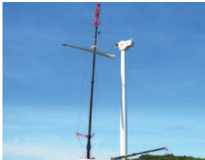
A turbine under construction
