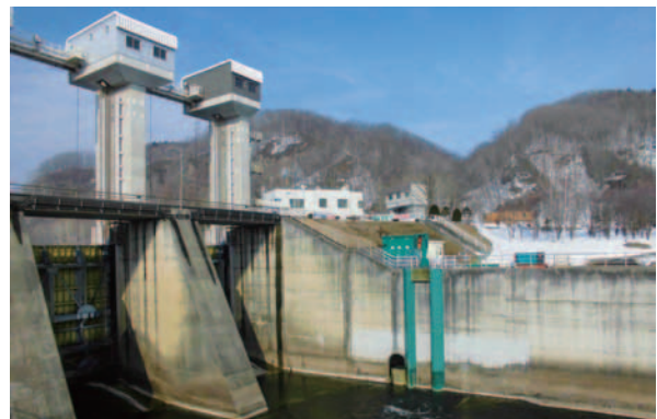
The Kuttari Power Station (Hokkaido)
