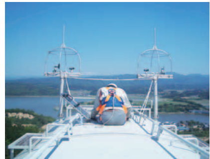
Maintenance work being performed on the nacelle of a wind turbine
