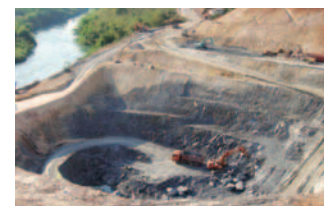
Foundation excavation work for the Thac Mo power station
