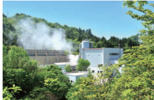
Onikobe Geothermal Power Station (Miyagi Prefecture)
