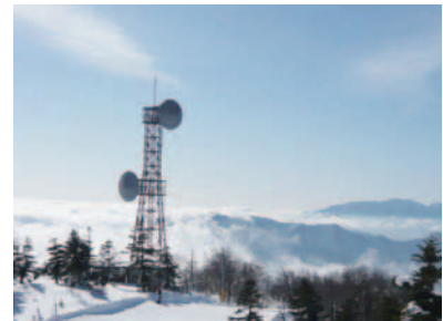
Takatsue Radio Relay Station (Fukushima Prefecture)
