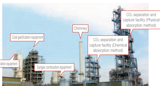
External view of EAGLE Pilot Plant test facility (Kitakyushu City)
