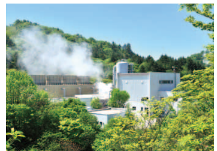
Onikobe Geothermal Power Station (Miyagi Prefecture)
