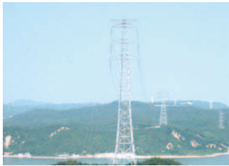
Honshu-Shikoku Interconnection (Okayama and Kagawa Prefecture) 500,000-volt transmission lines across the Seto Inland Sea to connect Honshu and Shikoku. These transmission lines are connected to backbone transmission lines in Honshu and Shikoku, contributing to stable electric supplies in western Japan.
