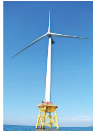
Embedded-type offshore wind power generation equipment (Kitakyushu city)
