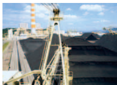
Matsushima Thermal Power Station coal yard
