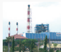
Tambak Lorok Power Station
