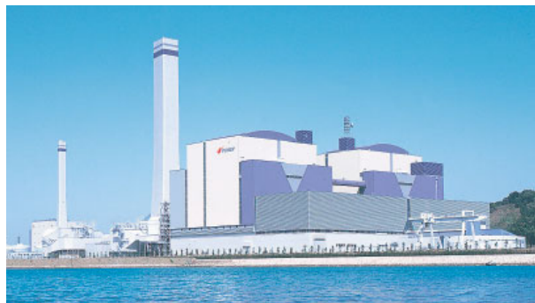
Tachibanawan Thermal Power Station (Tokushima Prefecture)
