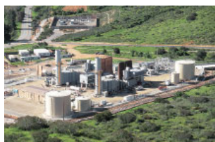
Orange Grove Power Station (U.S.A)
