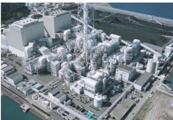
Matsuura Thermal Power Station (Nagasaki Prefecture)
