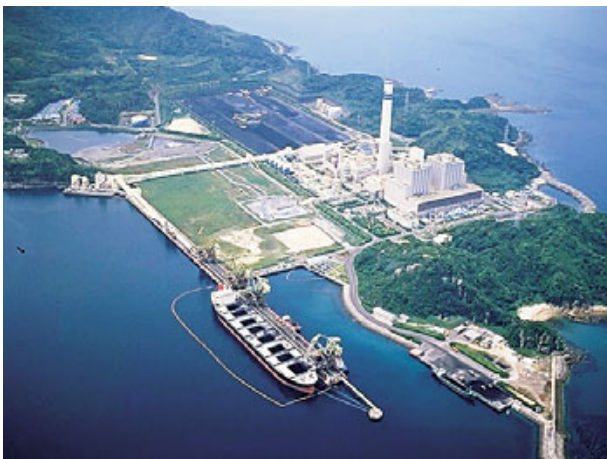
Matsushima Thermal Power Station (Nagasaki Prefecture)
