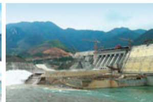
Son La Hydroelectric Power Station (Vietnam)
