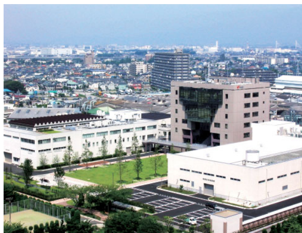
Technology Development Center Chigasaki Research Institute (Kanagawa Prefecture)
