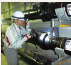
Patrolling the Honshi Interconnecting Line
