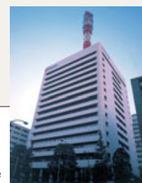
Steel telecommunications tower at the Head Office
