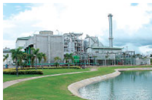
Roi-Et Biomass Power Station (Thailand)
