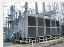
Inspecting a transformer
