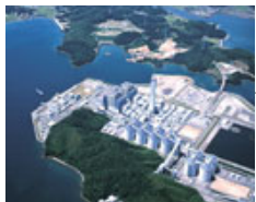
Tachibanawan Thermal Power Station
