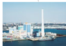
Isogo Thermal Power Station
