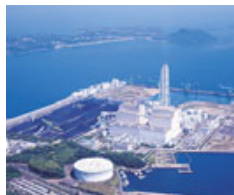
Matsuura Thermal Power Station
