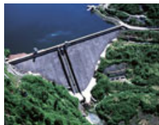
Okutadami Power Station
