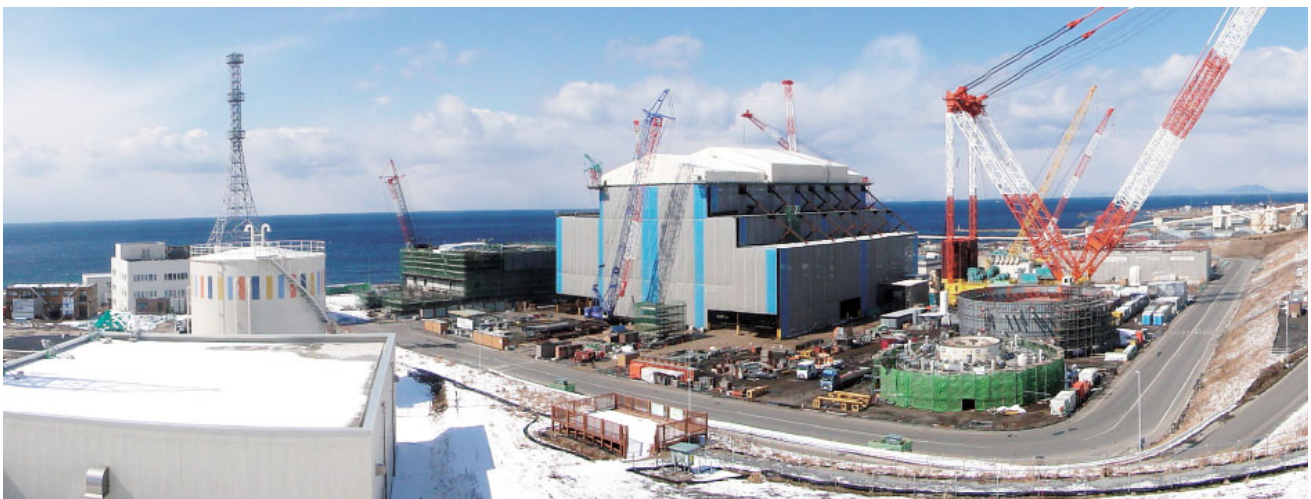
Status of construction of Ohma Nuclear Power Station (March 2011)
