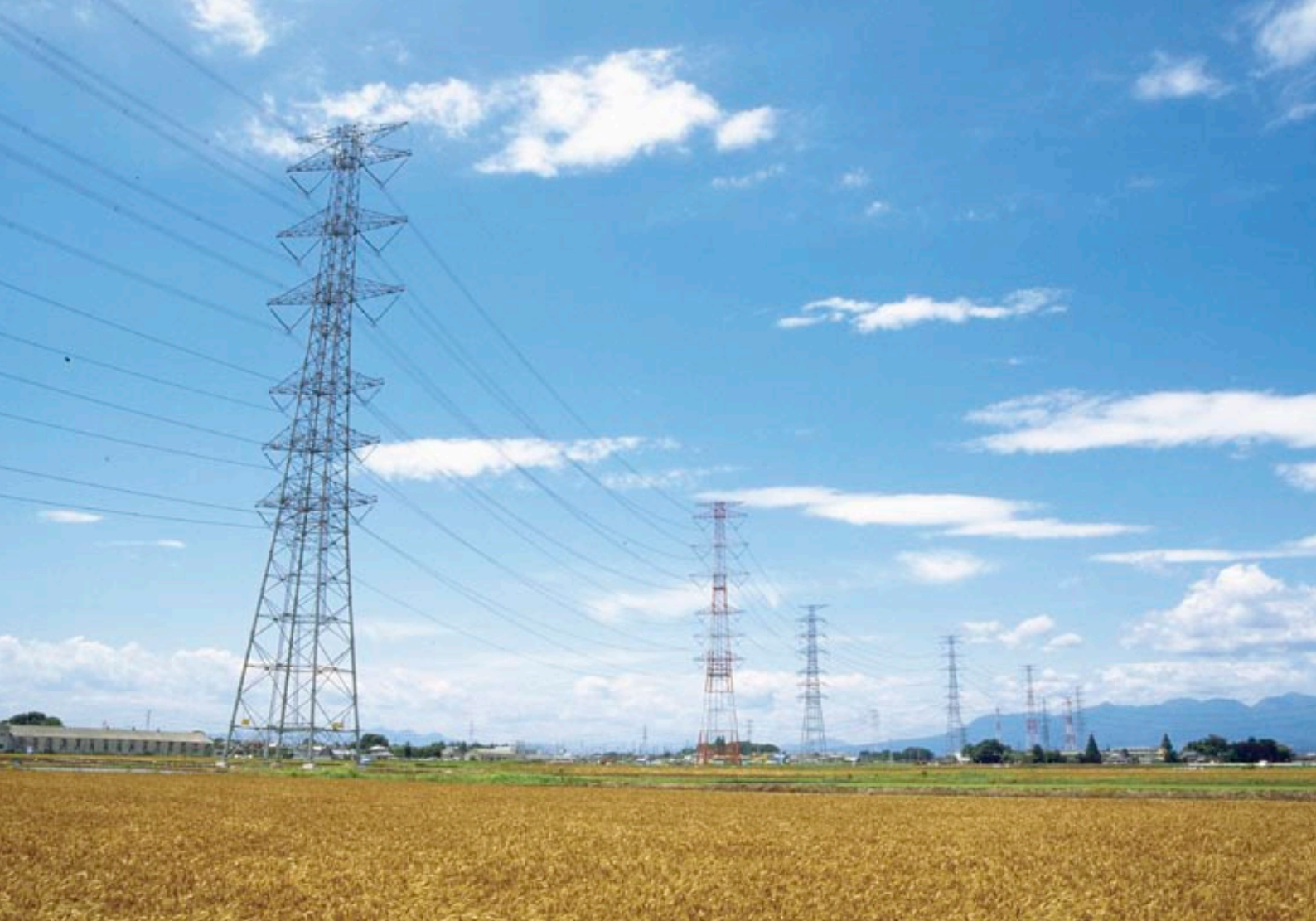
Tadami Main Transmission Line (Gunma Prefecture)
