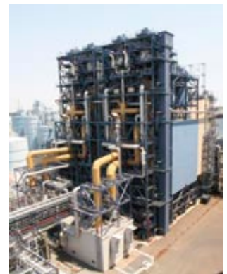
Dry-type desulfurization system at Isogo Thermal Power Station New No. 2 Unit (Yokohama)
